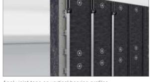
Apply joint tape on vertical bearing profiles
